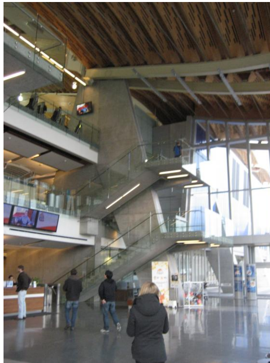
Figure 5 - Atrium Stairwell Surrounding Roof Buttress
