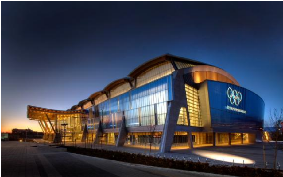
Figure 1 - The Richmond Olympic Oval [1]
