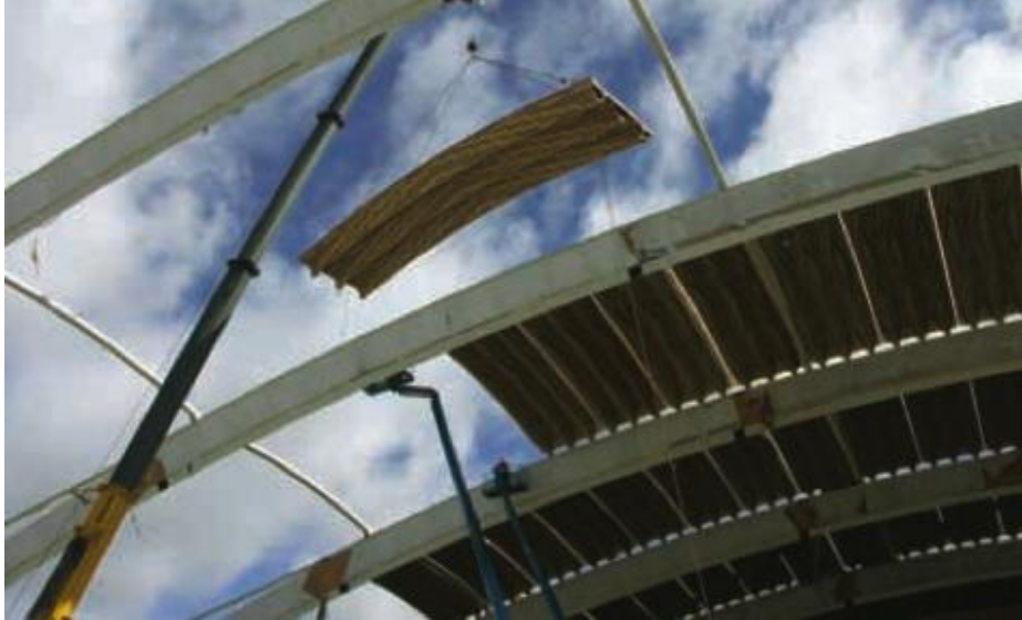
Figure 12 - Woodwave Panels Installed Between Composite V-Beams [3]
