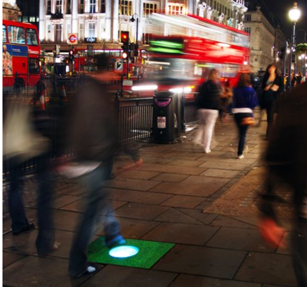
Figure 2: Installed Pavegen Tile
