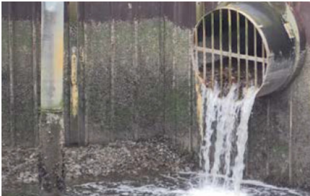
Image 8. Sewer outfall into the ocean 1 .
