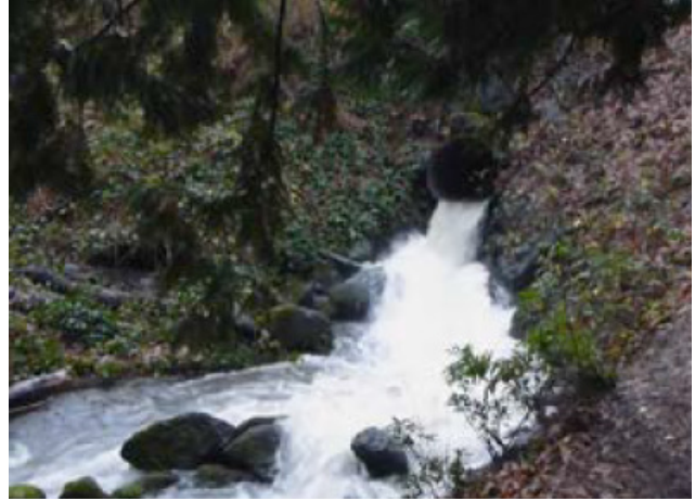
Image 7. Sewer outfall into a stream with fast flows 1 .
