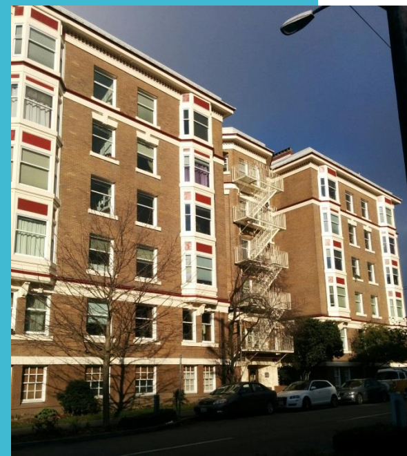
[Figure 12, East View, looking from Thurlow]
