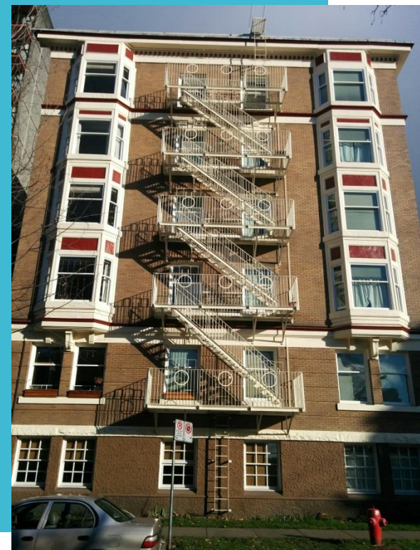
[Figure 13. East View, looking from Thurlow]
