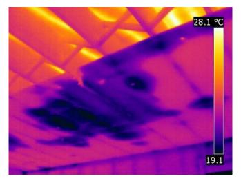
Figure 11. Moisture build-up in a ceiling. Image: Integrity Environmental Services.<sup>11</sup>
