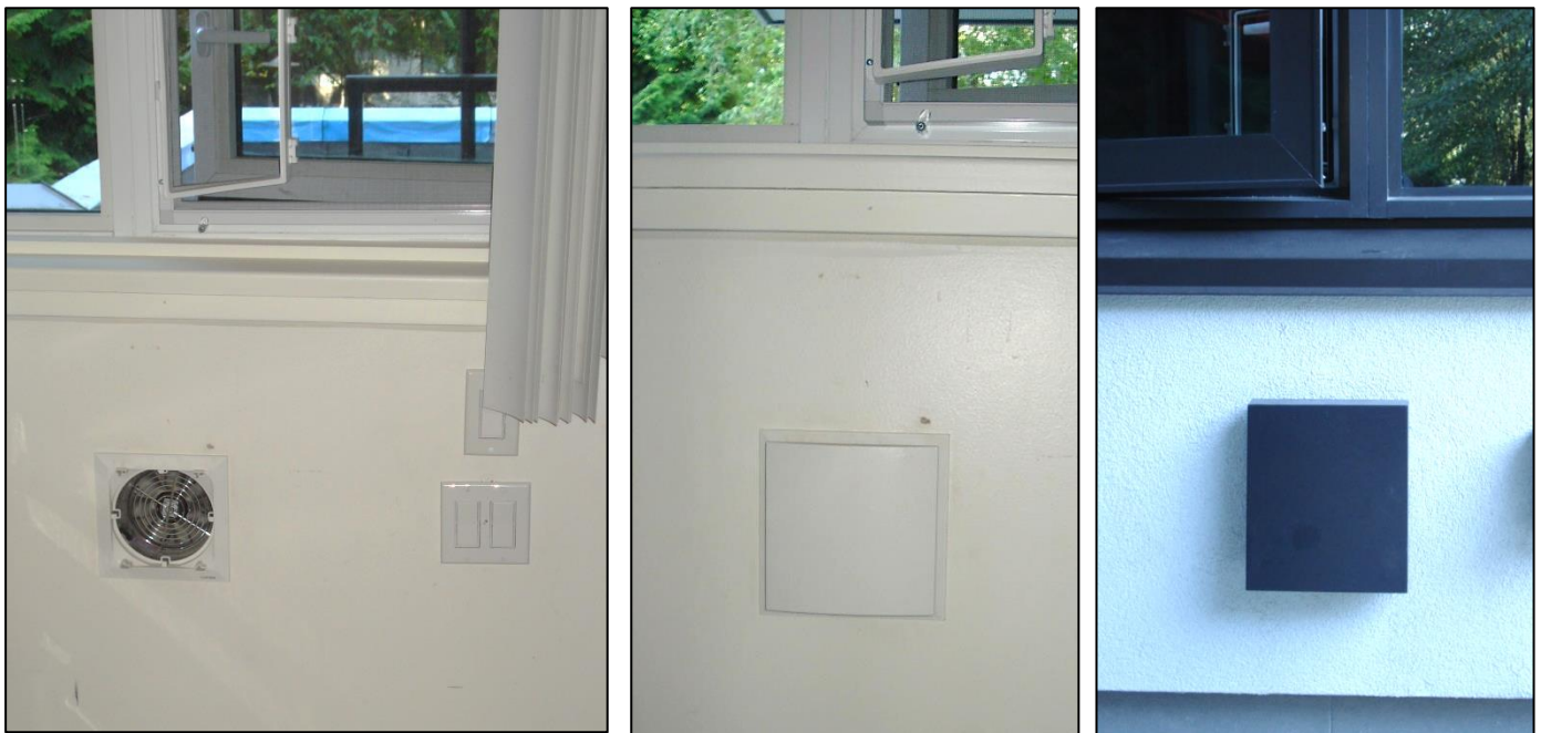
Pictures of the same Lunos e2 unit installed at a Concorde Place townhouse unit (from left to right):
