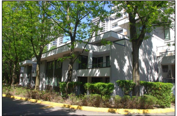
Front side of Concorde Place townhouse complex.
