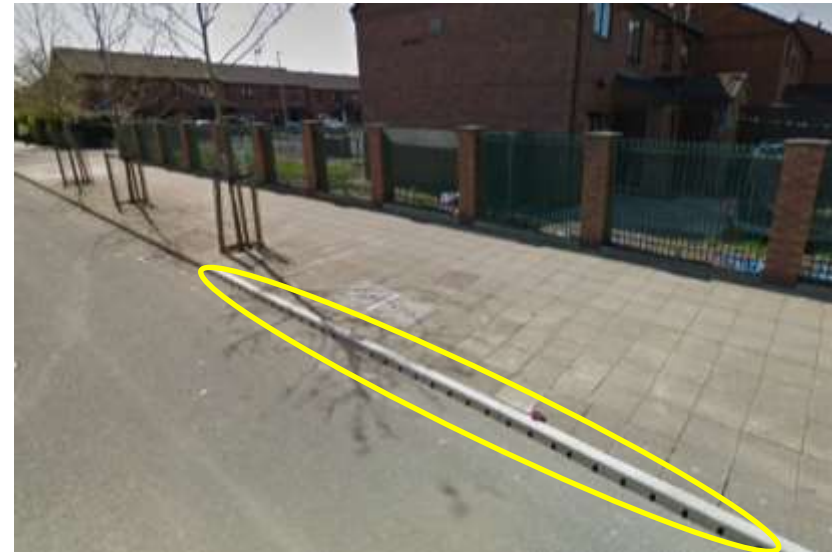
Figure 18: STT Curve Inlet System circled in yellow. Image source: Google Map data ©2018
