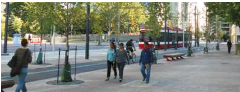
Figure 10: Silva Cells are used to support the Martin Goodman Bike Path while providing soil volume for the street trees along Queens Quay, which was reconstructed in 2014. Image source: Deep Root [48].
