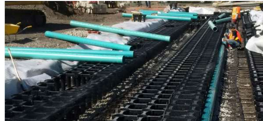
Figure 8: Thomson Family Park Soil Cell. Image source: Citygreen [37]
