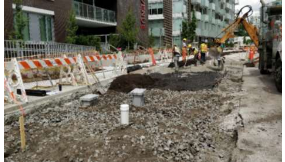
Structural soil during construction looking north
