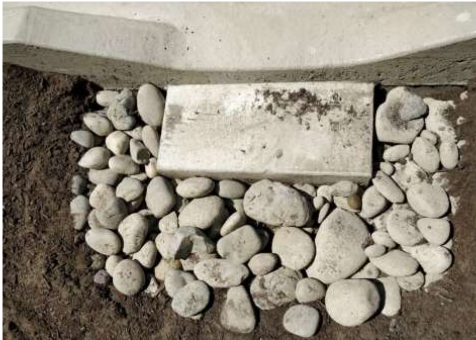
Figure 40: Bioswale inlet design
