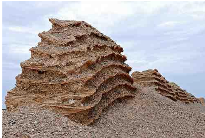
Figure 15: Great Wall of China – eroded rammed earth wall (Built 2500 years ago) 11
