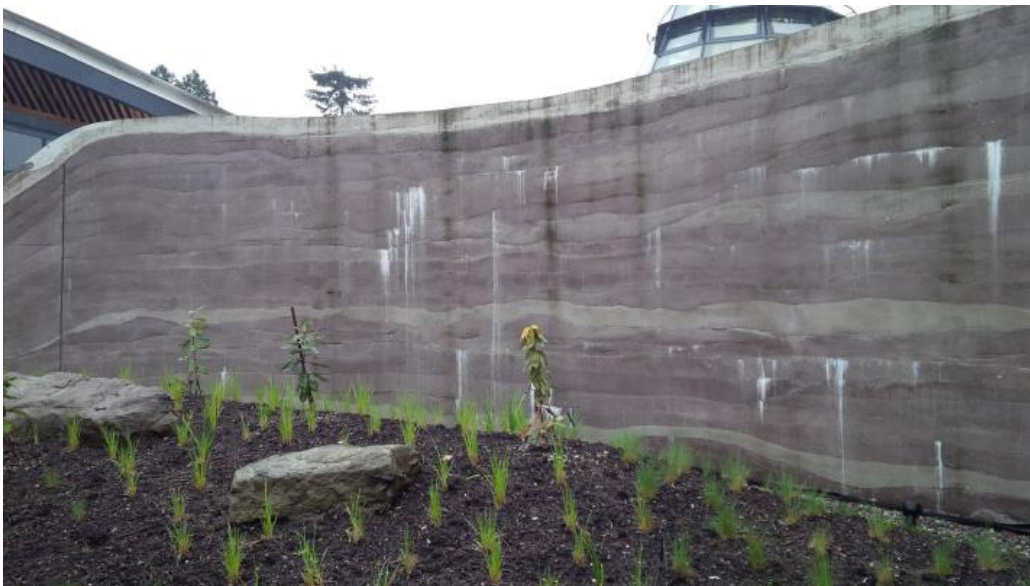
Figure 20: Efflorescence at cold joints in rammed earth wall, Van Dusen Botanical Garden 16
