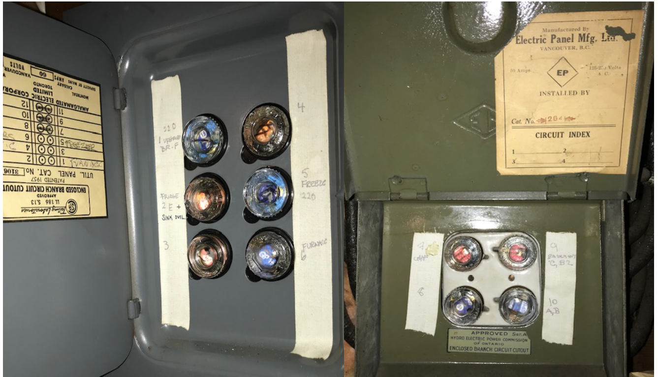
Figure 2:60-amp service panel
