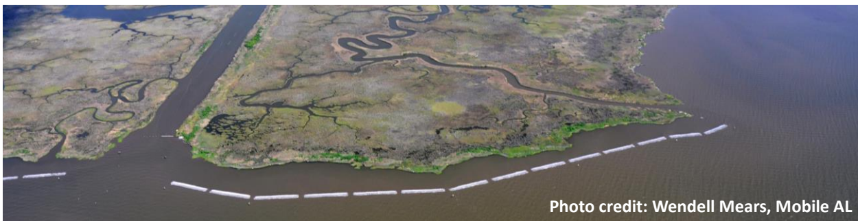
Figure 21. Straight on view of living shoreline breakwaters in Hancock County, MS (used with permission)
