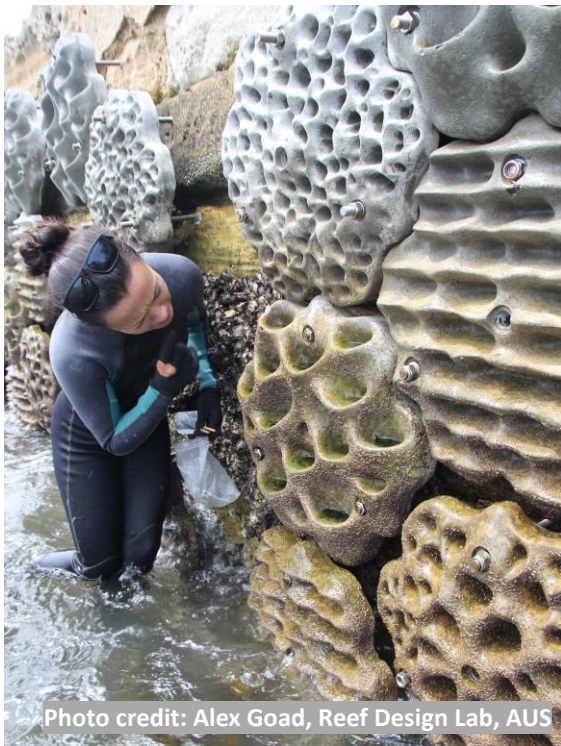
Figure 28. Closer look at the Living Seawall tiles (used with permission)
