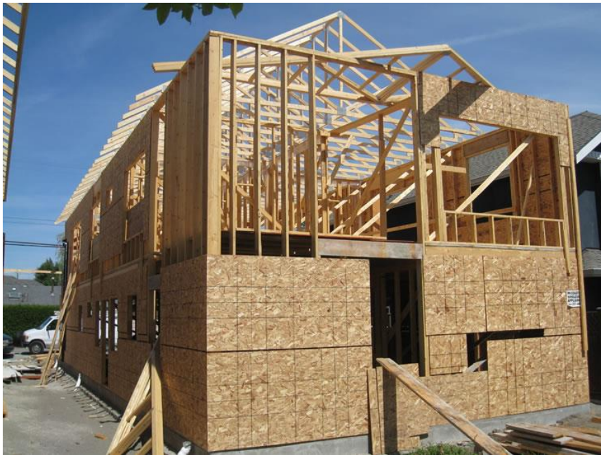
Figure 7. Oriented-strand board sheathing. Photo by NRCAN, 2020, via https://www.nrcan.gc.ca/our-natural-resources/forests-forestry/forest-industry-trade/forest-products-applications/taxonomy-wood-products/oriented-strand-board/15851
