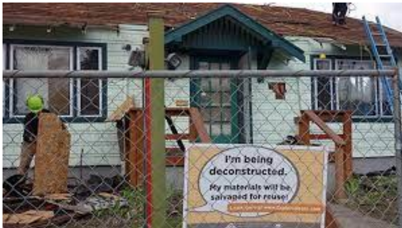
Figure 10. Hand deconstruction in Portland. Photo by Construction & Demolition Recycling, 2016, via https://www.cdrecycler.com/article/portland-oregon-deconstruction-ordinance/
