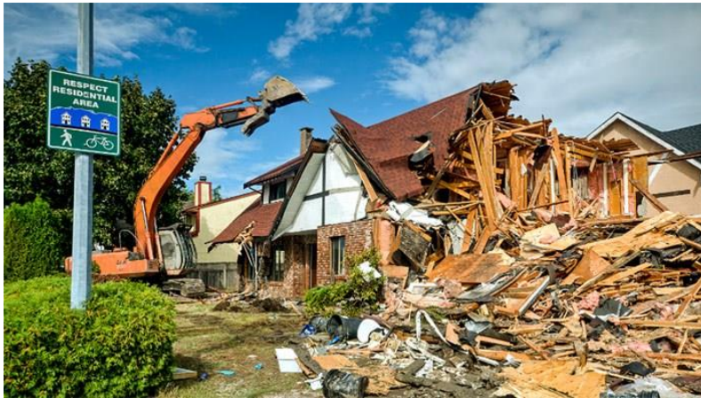
Figure 1. Vancouver demolition. Photo by Chung Chow, found via https://www.vancouverisawesome.com/vancouver-news/vancouver-demolition-teardown-study-1938266
