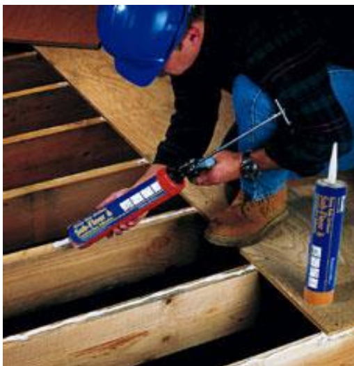
Figure 6. Applying sub-floor adhesive. Photo by Bostik Findley Inc., via https://www.adhesivesandsealants.com/doc/chem-calk-heavy-duty-urethane-construction-ad-0001
