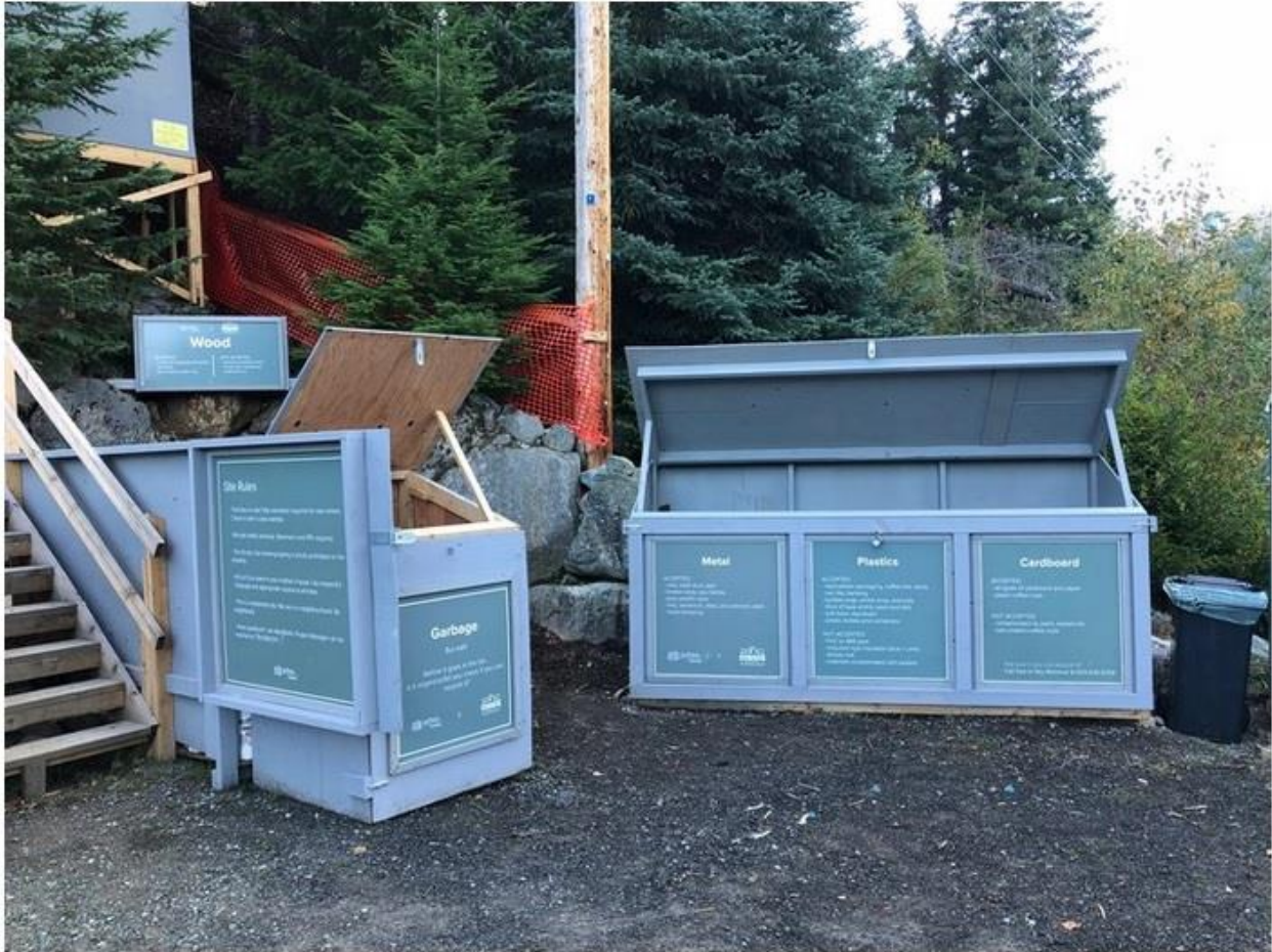
Figure 12. Sea to Sky on-site sorting station. Photo by Sea to Sky Removal, 2018, via https://www.seatoskyremoval.ca/sea-to-sky-removal-blog/2018/9/28/sea-to-sky-removal-interviews-adisa-homes-ltd-on-sustainable-waste-managment .
