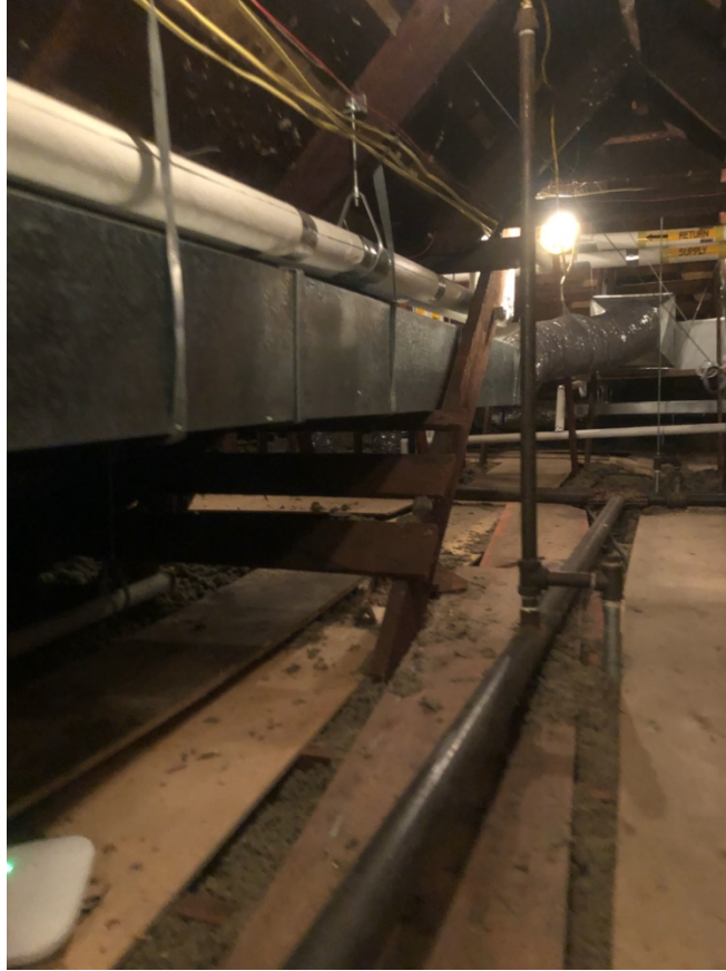
Fig.19 Distribution system in the attic
