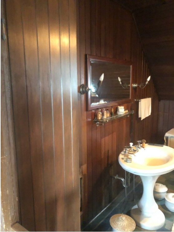
Fig.10 Hidden pipes in the second-floor bathroom
