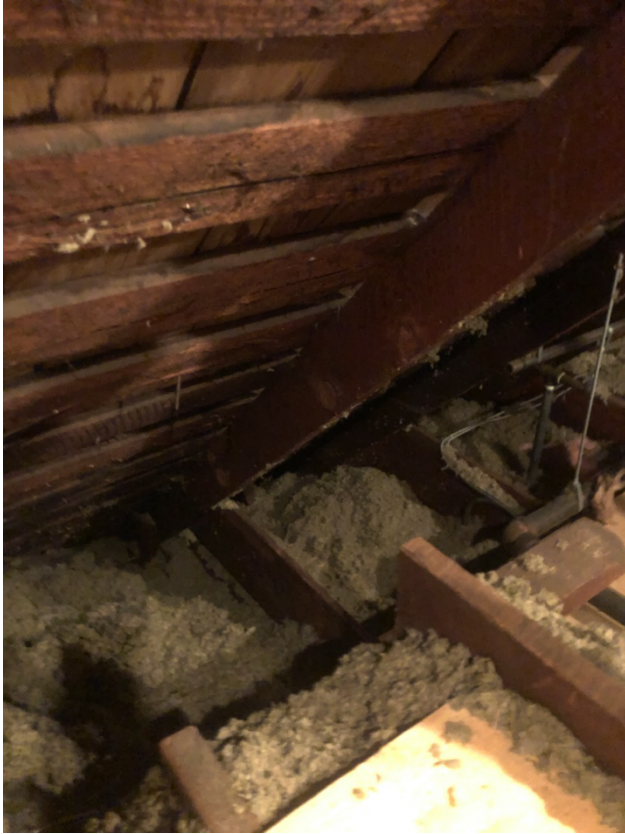
Fig.8 Blown-in cellulose insulation in the attic
