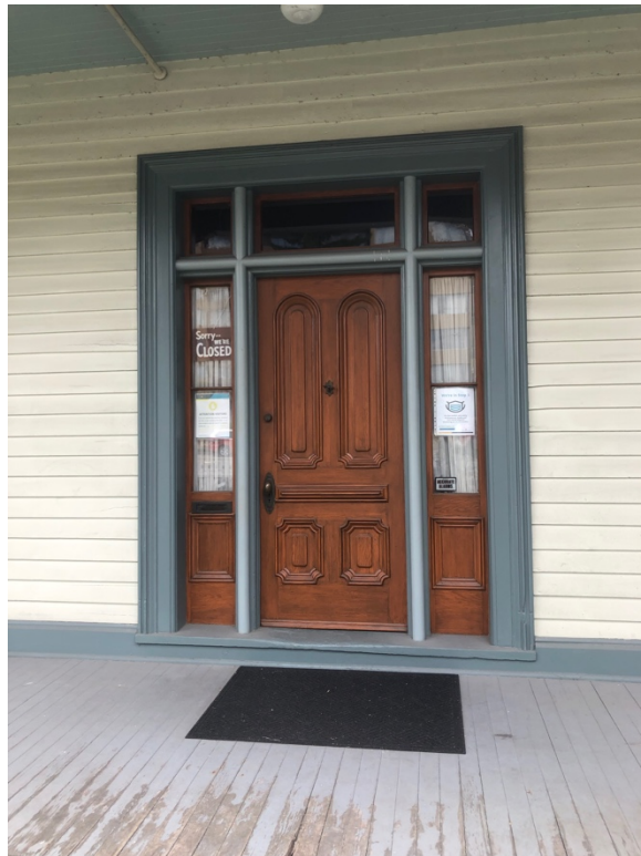
Fig.14 Original door on the front entrance
