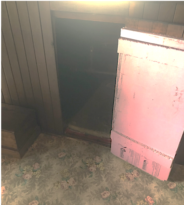
Fig.9 Batt insulation and foam board on the door
