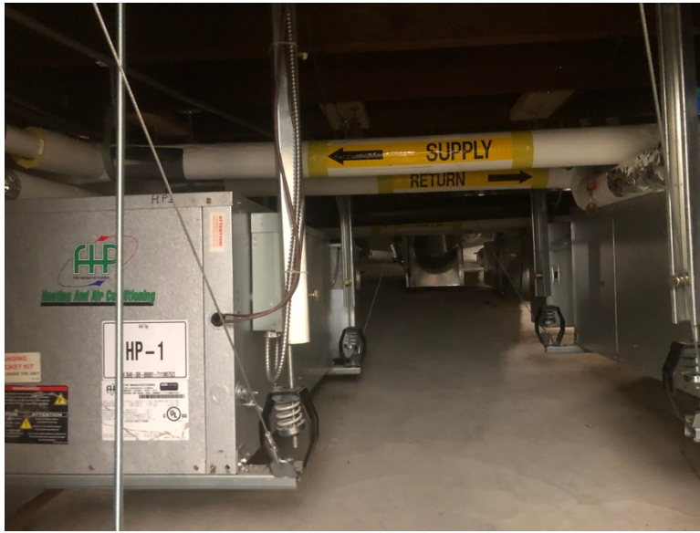
Fig.15 Distribution system in the crawl space
