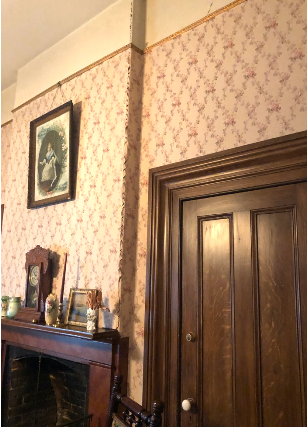
Fig.6 Wallpaper degradation
