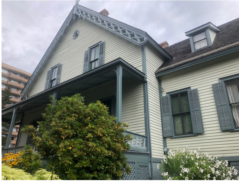
Fig.13 West side of the property
