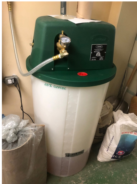
Fig.16 Buffer tank in the crawl space
