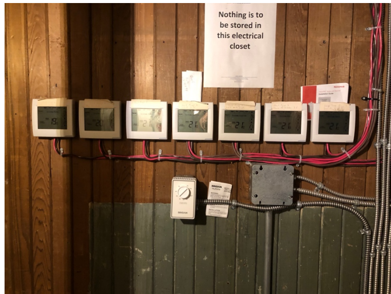
Fig.18 Thermostats located in a closet on the main floor
