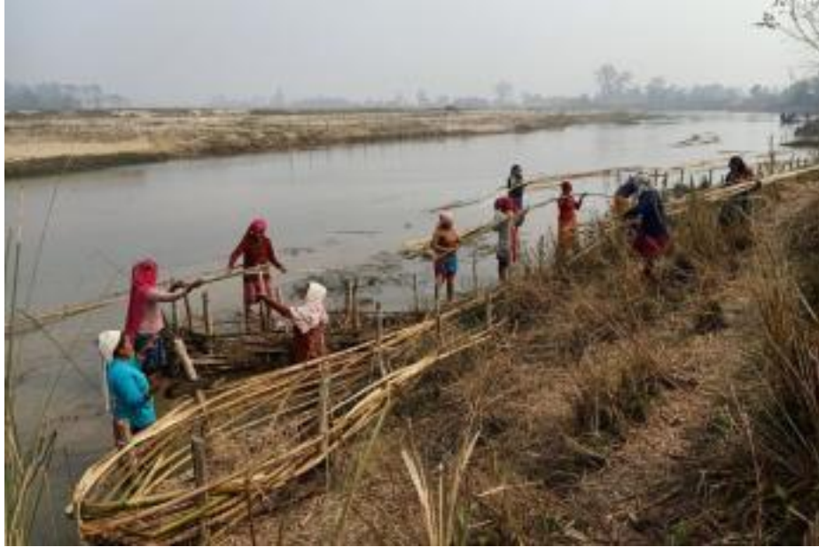
Fig 8. Women in Badabaika, Nepal build bamboo spurs as protection from floods. Source: Ojha (2021).
