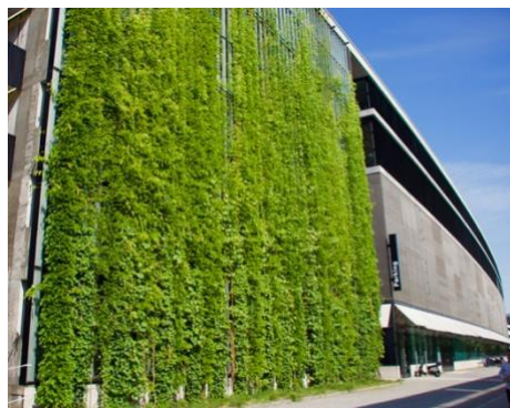
Figure 5 Cable supported green wall
