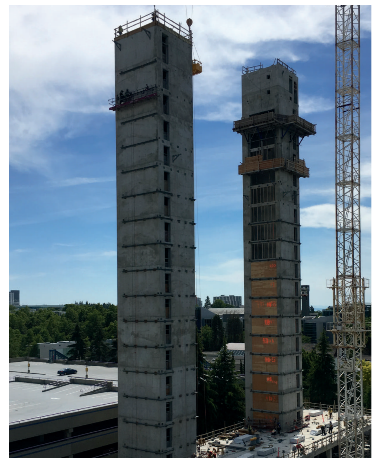
Construction of concrete cores (June 2016)
