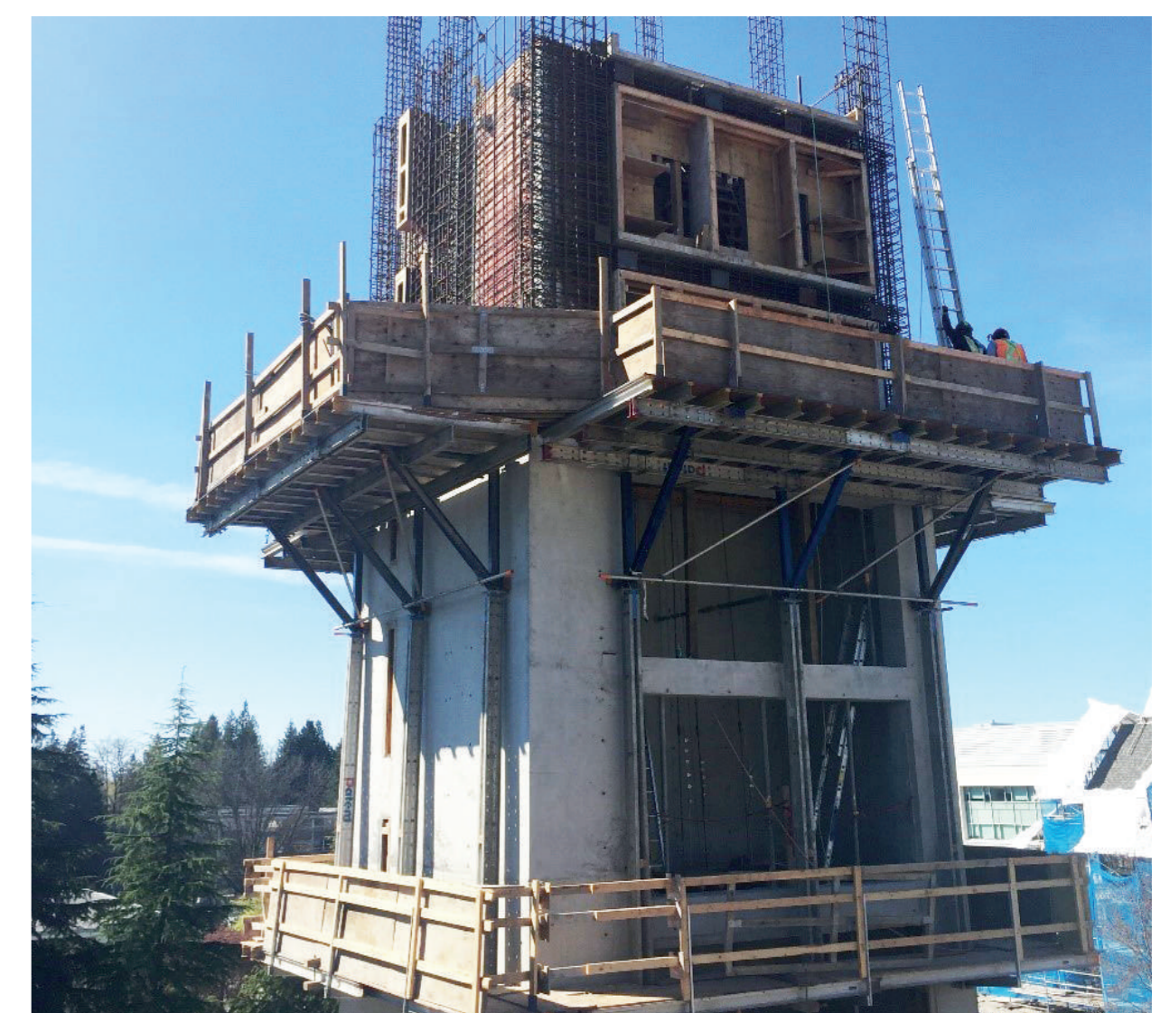
Actual concrete core under construction
