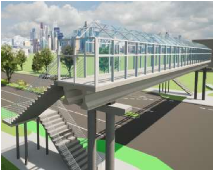
Figure 17 Bent Cap and Integrated Concrete Columns
