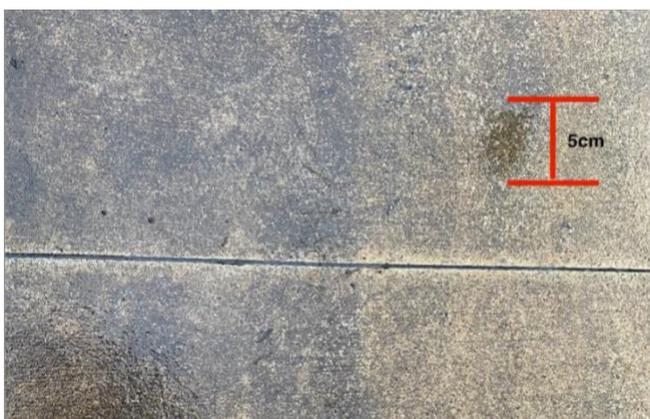
Figure 18. The photo of small ponding of 5 cm in length was taken on February 11<sup>th</sup>, 2024.
