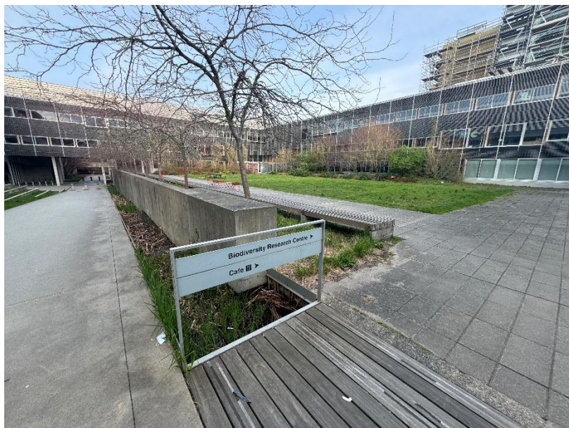
Figure 9. Beaty green roof, showing trimming of wetland vegetation in drainage channel on left.
