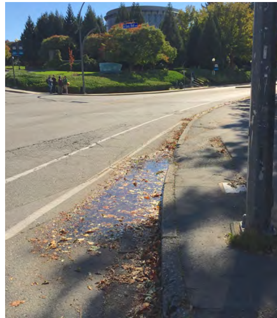
Figure 11: Ponding Along North Curb Alignment (Documented September 21, 2015)
